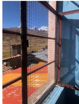
Our new scale and wire screens have been installed and positioned. Wire screens will help keep moisture out, while also preventing birds from shitting inside the building.
