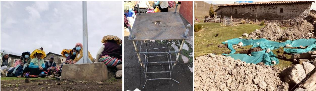
The main post sits on a solid concrete structure. There is a metal frame underneath (middle photo). In the image to the right, a lot of work has been done with an excavator we had to hire in order to make the Ground Rod. 3 wells of 2.60 meters deep have been dug.
