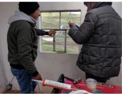
Installing a glass for the window to protect our generator from the harsh weather.
